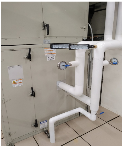
Figure 2: Server Room Cooling Coil
