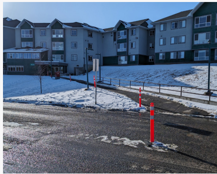
Nice delineator placement along the path for edge awareness from student housing to campus facilities.
