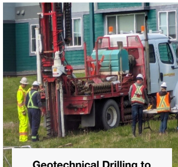
Geotechnical Drilling to determine sub-surface characteristics.
