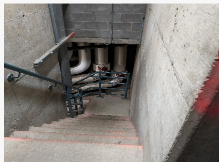
Painted stair ends & wall corner for visibility.
