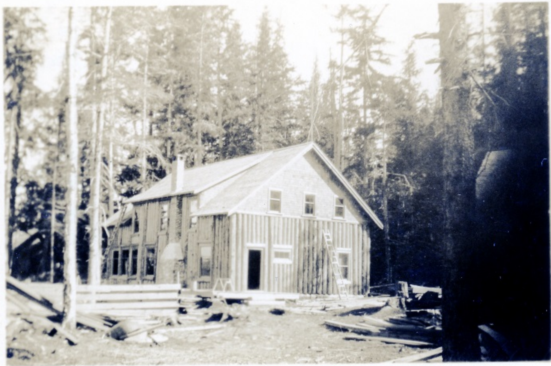
Lakeshore Lodge under construction. 1929. Johnstone Collection.
