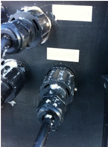
Figure 1. Radar cables attached to protected sockets on outside of pelican case
