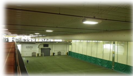
Energy retrofits at the Northern Sport Centre
