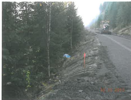
Photo 12 above: View of one of the new culverts at the site (this one is between C1 and C2 just above the first curve in the roadway). Note the use of rock armour on the bank and around the culvert inlet, and the improved ditch capacity. The inset shows a typical view of a flume installed below a culvert outlet (typical of new/repared culverts where discharge crosses a road fill embankment). Photo 13 upper middle: View looking along the roadway with final surface grading in progress. Note the insloped road surface profile which was developed as per design requirements. Note also the re-shaping of the road shoulder to a beveled configuration, along the outside margin of the new road surface. Photo 14 upper right: View looking easterly along the restored roadway at the slide area (red arrows). The culvert in the photo is C2, which was re-located just above the slide as part of the repair. The roadway was restored to its original width in the slide area and the ditch line was reinstated after construction as shown. Inset: View of the ditchline near culvert C3 just down slope/east of the slide repair. The seepage in the ditchline appeared after it was re-instated (the ditch had been temporarily infilled during slide repair). Photo 15 lower left: View of a small sinkhole erosion feature which opened up at the location of culvert C4 in the middle of the roadway. The inset shows a closeup view inside the sinkhole where one end of a culvert segment can be seen, indicating that there was a gap between two culvert pipes. Both the existing culverts C4 and C5 were exposed and repaired by Gibraltar, as clamps had not been used to secure the adjoining pipe segment together at either location. Photo 16 lower middle: View of the road shoulder and C9 culvert outlet after replacement of the old culvert, looking easterly towards the main QRRC building. Photo 17 lower right: View looking easterly along the upper road to the residence. Road grading and ditch improvement was in progress at the time the photo was taken. The inlet for the new C9 culvert is in the foreground of the photo. The stockpile of crushed aggregate in the photo was to be used to modify the road surface to direct more of the runoff from the upper road into the ditch and C9 culvert, rather than the previous condition where it flowed around the intersection and down towards the administration building.
