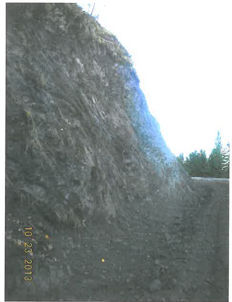
Photo 1 above: Preconstruction view looking west/upslope along the roadway segment adjoining the rock bluff. Note the obstructed sight lines at the road corner, lack of a ditch line/debris catchment area along the slope toe, and infilled/outwards leaning barrier elements. Photo 2 upper middle: view from a similar location after construction. The rock slope toe area was trimmed to establish a ditch/debris catchment area along the slope toe, and vegetation was removed from the lower part of the slope. Note the concrete guardrail blocks (photo centre) were lifted and re-seated on a low fill embankment. The window of gravel along the guardrail created during grading was removed after the photo was taken. Photo 3 upper right: closeup view of the east/downslope end of the rock slope toe area which was reconfigured by Gibraltar. Photo 4 lower left: View looking westerly "around the corner" at the west end of the rock outcrop area. Note the improved sight lines along the corner, and ditchline established at the slope toe. Photo 5 lower middle: View looking easterly/down the road, at the central part of the rock slope which was trimmed. Note the clearing/removal of vegetation above the crest of the cut slope. Ideally, small trees which become established in this area should be removed from time to time, to prevent them from growing to mature size to the stage they may become a hazard to road users.
