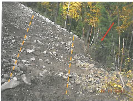
Photo 6 above: View of the temporary access trail under construction, during initial preparation for slide repair. As the temporary slope height exceeded 6 m, a written "safe entry" protocol was developed by AMEC under which Gibraltar's staff was conditionally granted access to work in the excavation. The large boulders in the photo were scavenged from the existing embankment fill and were incorporated into the lower "stack wall" part of the embankment repair. The inset view shows the temporary stockpile of rip rap armour which was obtained from Mt. Polley. Photo 7 upper middle: View looking upslope in the scour channel developed below the slide, at the toe of the new embankment. The boulders were placed individually on a prepared base and interlocked at a nominal 40-45° slope. The inset view shows the scale of some of the larger rip rap blocks placed at the slide toe. Photo 8 upper right: Panoramic view looking downslope at the former slide area, from the restored road shoulder. The dashed line marks the approximate transition from larger placed rip rap, and more variably sized angular rock (both from Mt. Polley and from the rock slope area at the site). The inset is a closeup view of the flow channel below the slide. Some rock chunks came loose during placement, and came to rest a short distance downslope in an area of irregular bedrock exposed in the debris channel created below the slide zone. The rocks are interlocked and are considered to be stable. Photo 9 lower left: View looking downslope across the restored road fill embankment. The dashed lines mark the approximate location of the temporary access trail. The red arrow points to the approximate location of loose fills dispersed downslope into the forest during trail construction (see Photo 10). Photo 10 lower middle: View looking easterly across the fill materials on the ground surface downslope from the temporary access trail. The slope of the fill is approximately 38°. Photo 11 lower right: Panoramic view looking up/westerly along the restored roadway and fill embankment area at the slide repair site.
