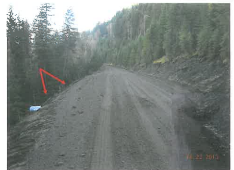
Photo 12 above: View of one of the new culverts at the site (this one is between C1 and C2 just above the first curve in the roadway). Note the use of rock armour on the bank and around the culvert inlet, and the improved ditch capacity. The inset shows a typical view of a flume installed below a culvert outlet (typical of new/repared culverts where discharge crosses a road fill embankment). Photo 13 upper middle: View looking along the roadway with final surface grading in progress. Note the insloped road surface profile which was developed as per design requirements. Note also the re-shaping of the road shoulder to a beveled configuration, along the outside margin of the new road surface. Photo 14 upper right: View looking easterly along the restored roadway at the slide area (red arrows). The culvert in the photo is C2, which was re-located just above the slide as part of the repair. The roadway was restored to its original width in the slide area and the ditch line was reinstated after construction as shown. Inset: View of the ditchline near culvert C3 just down slope/east of the slide repair. The seepage in the ditchline appeared after it was re-instated (the ditch had been temporarily infilled during slide repair). Photo 15 lower left: View of a small sinkhole erosion feature which opened up at the location of culvert C4 in the middle of the roadway. The inset shows a closeup view inside the sinkhole where one end of a culvert segment can be seen, indicating that there was a gap between two culvert pipes. Both the existing culverts C4 and C5 were exposed and repaired by Gibraltar, as clamps had not been used to secure the adjoining pipe segment together at either location. Photo 16 lower middle: View of the road shoulder and C9 culvert outlet after replacement of the old culvert, looking easterly towards the main QRRC building. Photo 17 lower right: View looking easterly along the upper road to the residence. Road grading and ditch improvement was in progress at the time the photo was taken. The inlet for the new C9 culvert is in the foreground of the photo. The stockpile of crushed aggregate in the photo was to be used to modify the road surface to direct more of the runoff from the upper road into the ditch and C9 culvert, rather than the previous condition where it flowed around the intersection and down towards the administration building.
