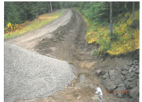
Photo 12 above: View of one of the new culverts at the site (this one is between C1 and C2 just above the first curve in the roadway). Note the use of rock armour on the bank and around the culvert inlet, and the improved ditch capacity. The inset shows a typical view of a flume installed below a culvert outlet (typical of new/repared culverts where discharge crosses a road fill embankment). Photo 13 upper middle: View looking along the roadway with final surface grading in progress. Note the insloped road surface profile which was developed as per design requirements. Note also the re-shaping of the road shoulder to a beveled configuration, along the outside margin of the new road surface. Photo 14 upper right: View looking easterly along the restored roadway at the slide area (red arrows). The culvert in the photo is C2, which was re-located just above the slide as part of the repair. The roadway was restored to its original width in the slide area and the ditch line was reinstated after construction as shown. Inset: View of the ditchline near culvert C3 just down slope/east of the slide repair. The seepage in the ditchline appeared after it was re-instated (the ditch had been temporarily infilled during slide repair). Photo 15 lower left: View of a small sinkhole erosion feature which opened up at the location of culvert C4 in the middle of the roadway. The inset shows a closeup view inside the sinkhole where one end of a culvert segment can be seen, indicating that there was a gap between two culvert pipes. Both the existing culverts C4 and C5 were exposed and repaired by Gibraltar, as clamps had not been used to secure the adjoining pipe segment together at either location. Photo 16 lower middle: View of the road shoulder and C9 culvert outlet after replacement of the old culvert, looking easterly towards the main QRRC building. Photo 17 lower right: View looking easterly along the upper road to the residence. Road grading and ditch improvement was in progress at the time the photo was taken. The inlet for the new C9 culvert is in the foreground of the photo. The stockpile of crushed aggregate in the photo was to be used to modify the road surface to direct more of the runoff from the upper road into the ditch and C9 culvert, rather than the previous condition where it flowed around the intersection and down towards the administration building.
