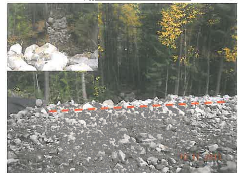
Photo 6 above: View of the temporary access trail under construction, during initial preparation for slide repair. As the temporary slope height exceeded 6 m, a written "safe entry" protocol was developed by AMEC under which Gibraltar's staff was conditionally granted access to work in the excavation. The large boulders in the photo were scavenged from the existing embankment fill and were incorporated into the lower "stack wall" part of the embankment repair. The inset view shows the temporary stockpile of rip rap armour which was obtained from Mt. Polley. Photo 7 upper middle: View looking upslope in the scour channel developed below the slide, at the toe of the new embankment. The boulders were placed individually on a prepared base and interlocked at a nominal 40-45° slope. The inset view shows the scale of some of the larger rip rap blocks placed at the slide toe. Photo 8 upper right: Panoramic view looking downslope at the former slide area, from the restored road shoulder. The dashed line marks the approximate transition from larger placed rip rap, and more variably sized angular rock (both from Mt. Polley and from the rock slope area at the site). The inset is a closeup view of the flow channel below the slide. Some rock chunks came loose during placement, and came to rest a short distance downslope in an area of irregular bedrock exposed in the debris channel created below the slide zone. The rocks are interlocked and are considered to be stable. Photo 9 lower left: View looking downslope across the restored road fill embankment. The dashed lines mark the approximate location of the temporary access trail. The red arrow points to the approximate location of loose fills dispersed downslope into the forest during trail construction (see Photo 10). Photo 10 lower middle: View looking easterly across the fill materials on the ground surface downslope from the temporary access trail. The slope of the fill is approximately 38°. Photo 11 lower right: Panoramic view looking up/westerly along the restored roadway and fill embankment area at the slide repair site.
