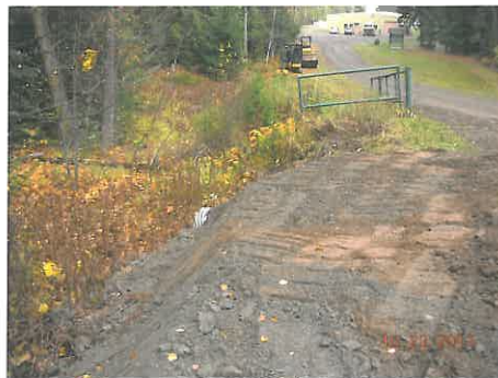
Photo 12 above: View of one of the new culverts at the site (this one is between C1 and C2 just above the first curve in the roadway). Note the use of rock armour on the bank and around the culvert inlet, and the improved ditch capacity. The inset shows a typical view of a flume installed below a culvert outlet (typical of new/repared culverts where discharge crosses a road fill embankment). Photo 13 upper middle: View looking along the roadway with final surface grading in progress. Note the insloped road surface profile which was developed as per design requirements. Note also the re-shaping of the road shoulder to a beveled configuration, along the outside margin of the new road surface. Photo 14 upper right: View looking easterly along the restored roadway at the slide area (red arrows). The culvert in the photo is C2, which was re-located just above the slide as part of the repair. The roadway was restored to its original width in the slide area and the ditch line was reinstated after construction as shown. Inset: View of the ditchline near culvert C3 just down slope/east of the slide repair. The seepage in the ditchline appeared after it was re-instated (the ditch had been temporarily infilled during slide repair). Photo 15 lower left: View of a small sinkhole erosion feature which opened up at the location of culvert C4 in the middle of the roadway. The inset shows a closeup view inside the sinkhole where one end of a culvert segment can be seen, indicating that there was a gap between two culvert pipes. Both the existing culverts C4 and C5 were exposed and repaired by Gibraltar, as clamps had not been used to secure the adjoining pipe segment together at either location. Photo 16 lower middle: View of the road shoulder and C9 culvert outlet after replacement of the old culvert, looking easterly towards the main QRRC building. Photo 17 lower right: View looking easterly along the upper road to the residence. Road grading and ditch improvement was in progress at the time the photo was taken. The inlet for the new C9 culvert is in the foreground of the photo. The stockpile of crushed aggregate in the photo was to be used to modify the road surface to direct more of the runoff from the upper road into the ditch and C9 culvert, rather than the previous condition where it flowed around the intersection and down towards the administration building.
