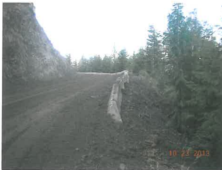
Photo 1 above: Preconstruction view looking west/upslope along the roadway segment adjoining the rock bluff. Note the obstructed sight lines at the road corner, lack of a ditch line/debris catchment area along the slope toe, and infilled/outwards leaning barrier elements. Photo 2 upper middle: view from a similar location after construction. The rock slope toe area was trimmed to establish a ditch/debris catchment area along the slope toe, and vegetation was removed from the lower part of the slope. Note the concrete guardrail blocks (photo centre) were lifted and re-seated on a low fill embankment. The window of gravel along the guardrail created during grading was removed after the photo was taken. Photo 3 upper right: closeup view of the east/downslope end of the rock slope toe area which was reconfigured by Gibraltar. Photo 4 lower left: View looking westerly "around the corner" at the west end of the rock outcrop area. Note the improved sight lines along the corner, and ditchline established at the slope toe. Photo 5 lower middle: View looking easterly/down the road, at the central part of the rock slope which was trimmed. Note the clearing/removal of vegetation above the crest of the cut slope. Ideally, small trees which become established in this area should be removed from time to time, to prevent them from growing to mature size to the stage they may become a hazard to road users.
