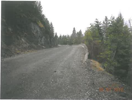
Photo 1 above: Preconstruction view looking west/upslope along the roadway segment adjoining the rock bluff. Note the obstructed sight lines at the road corner, lack of a ditch line/debris catchment area along the slope toe, and infilled/outwards leaning barrier elements. Photo 2 upper middle: view from a similar location after construction. The rock slope toe area was trimmed to establish a ditch/debris catchment area along the slope toe, and vegetation was removed from the lower part of the slope. Note the concrete guardrail blocks (photo centre) were lifted and re-seated on a low fill embankment. The window of gravel along the guardrail created during grading was removed after the photo was taken. Photo 3 upper right: closeup view of the east/downslope end of the rock slope toe area which was reconfigured by Gibraltar. Photo 4 lower left: View looking westerly "around the corner" at the west end of the rock outcrop area. Note the improved sight lines along the corner, and ditchline established at the slope toe. Photo 5 lower middle: View looking easterly/down the road, at the central part of the rock slope which was trimmed. Note the clearing/removal of vegetation above the crest of the cut slope. Ideally, small trees which become established in this area should be removed from time to time, to prevent them from growing to mature size to the stage they may become a hazard to road users.
