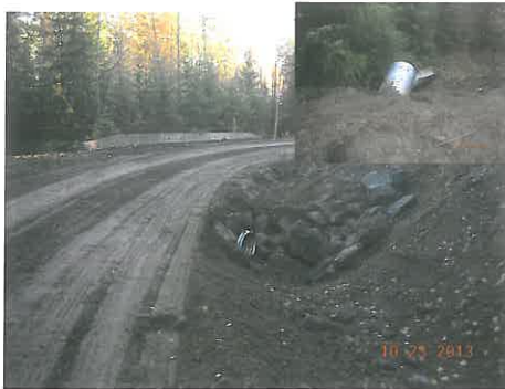
Photo 12 above: View of one of the new culverts at the site (this one is between C1 and C2 just above the first curve in the roadway). Note the use of rock armour on the bank and around the culvert inlet, and the improved ditch capacity. The inset shows a typical view of a flume installed below a culvert outlet (typical of new/repared culverts where discharge crosses a road fill embankment). Photo 13 upper middle: View looking along the roadway with final surface grading in progress. Note the insloped road surface profile which was developed as per design requirements. Note also the re-shaping of the road shoulder to a beveled configuration, along the outside margin of the new road surface. Photo 14 upper right: View looking easterly along the restored roadway at the slide area (red arrows). The culvert in the photo is C2, which was re-located just above the slide as part of the repair. The roadway was restored to its original width in the slide area and the ditch line was reinstated after construction as shown. Inset: View of the ditchline near culvert C3 just down slope/east of the slide repair. The seepage in the ditchline appeared after it was re-instated (the ditch had been temporarily infilled during slide repair). Photo 15 lower left: View of a small sinkhole erosion feature which opened up at the location of culvert C4 in the middle of the roadway. The inset shows a closeup view inside the sinkhole where one end of a culvert segment can be seen, indicating that there was a gap between two culvert pipes. Both the existing culverts C4 and C5 were exposed and repaired by Gibraltar, as clamps had not been used to secure the adjoining pipe segment together at either location. Photo 16 lower middle: View of the road shoulder and C9 culvert outlet after replacement of the old culvert, looking easterly towards the main QRRC building. Photo 17 lower right: View looking easterly along the upper road to the residence. Road grading and ditch improvement was in progress at the time the photo was taken. The inlet for the new C9 culvert is in the foreground of the photo. The stockpile of crushed aggregate in the photo was to be used to modify the road surface to direct more of the runoff from the upper road into the ditch and C9 culvert, rather than the previous condition where it flowed around the intersection and down towards the administration building.
