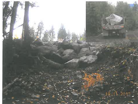
Photo 6 above: View of the temporary access trail under construction, during initial preparation for slide repair. As the temporary slope height exceeded 6 m, a written "safe entry" protocol was developed by AMEC under which Gibraltar's staff was conditionally granted access to work in the excavation. The large boulders in the photo were scavenged from the existing embankment fill and were incorporated into the lower "stack wall" part of the embankment repair. The inset view shows the temporary stockpile of rip rap armour which was obtained from Mt. Polley. Photo 7 upper middle: View looking upslope in the scour channel developed below the slide, at the toe of the new embankment. The boulders were placed individually on a prepared base and interlocked at a nominal 40-45° slope. The inset view shows the scale of some of the larger rip rap blocks placed at the slide toe. Photo 8 upper right: Panoramic view looking downslope at the former slide area, from the restored road shoulder. The dashed line marks the approximate transition from larger placed rip rap, and more variably sized angular rock (both from Mt. Polley and from the rock slope area at the site). The inset is a closeup view of the flow channel below the slide. Some rock chunks came loose during placement, and came to rest a short distance downslope in an area of irregular bedrock exposed in the debris channel created below the slide zone. The rocks are interlocked and are considered to be stable. Photo 9 lower left: View looking downslope across the restored road fill embankment. The dashed lines mark the approximate location of the temporary access trail. The red arrow points to the approximate location of loose fills dispersed downslope into the forest during trail construction (see Photo 10). Photo 10 lower middle: View looking easterly across the fill materials on the ground surface downslope from the temporary access trail. The slope of the fill is approximately 38°. Photo 11 lower right: Panoramic view looking up/westerly along the restored roadway and fill embankment area at the slide repair site.
