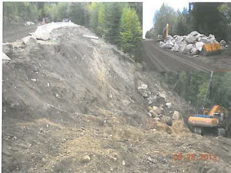
Photo 6 above: View of the temporary access trail under construction, during initial preparation for slide repair. As the temporary slope height exceeded 6 m, a written "safe entry" protocol was developed by AMEC under which Gibraltar's staff was conditionally granted access to work in the excavation. The large boulders in the photo were scavenged from the existing embankment fill and were incorporated into the lower "stack wall" part of the embankment repair. The inset view shows the temporary stockpile of rip rap armour which was obtained from Mt. Polley. Photo 7 upper middle: View looking upslope in the scour channel developed below the slide, at the toe of the new embankment. The boulders were placed individually on a prepared base and interlocked at a nominal 40-45° slope. The inset view shows the scale of some of the larger rip rap blocks placed at the slide toe. Photo 8 upper right: Panoramic view looking downslope at the former slide area, from the restored road shoulder. The dashed line marks the approximate transition from larger placed rip rap, and more variably sized angular rock (both from Mt. Polley and from the rock slope area at the site). The inset is a closeup view of the flow channel below the slide. Some rock chunks came loose during placement, and came to rest a short distance downslope in an area of irregular bedrock exposed in the debris channel created below the slide zone. The rocks are interlocked and are considered to be stable. Photo 9 lower left: View looking downslope across the restored road fill embankment. The dashed lines mark the approximate location of the temporary access trail. The red arrow points to the approximate location of loose fills dispersed downslope into the forest during trail construction (see Photo 10). Photo 10 lower middle: View looking easterly across the fill materials on the ground surface downslope from the temporary access trail. The slope of the fill is approximately 38°. Photo 11 lower right: Panoramic view looking up/westerly along the restored roadway and fill embankment area at the slide repair site.
