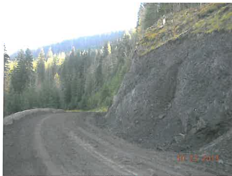
Photo 1 above: Preconstruction view looking west/upslope along the roadway segment adjoining the rock bluff. Note the obstructed sight lines at the road corner, lack of a ditch line/debris catchment area along the slope toe, and infilled/outwards leaning barrier elements. Photo 2 upper middle: view from a similar location after construction. The rock slope toe area was trimmed to establish a ditch/debris catchment area along the slope toe, and vegetation was removed from the lower part of the slope. Note the concrete guardrail blocks (photo centre) were lifted and re-seated on a low fill embankment. The window of gravel along the guardrail created during grading was removed after the photo was taken. Photo 3 upper right: closeup view of the east/downslope end of the rock slope toe area which was reconfigured by Gibraltar. Photo 4 lower left: View looking westerly "around the corner" at the west end of the rock outcrop area. Note the improved sight lines along the corner, and ditchline established at the slope toe. Photo 5 lower middle: View looking easterly/down the road, at the central part of the rock slope which was trimmed. Note the clearing/removal of vegetation above the crest of the cut slope. Ideally, small trees which become established in this area should be removed from time to time, to prevent them from growing to mature size to the stage they may become a hazard to road users.
