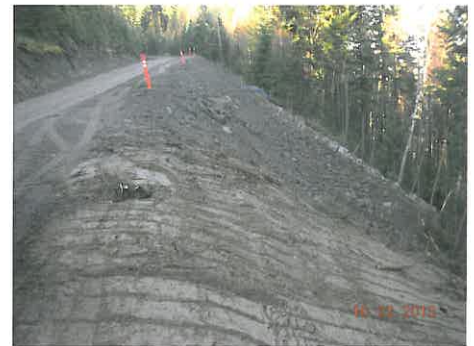
Photo 6 above: View of the temporary access trail under construction, during initial preparation for slide repair. As the temporary slope height exceeded 6 m, a written "safe entry" protocol was developed by AMEC under which Gibraltar's staff was conditionally granted access to work in the excavation. The large boulders in the photo were scavenged from the existing embankment fill and were incorporated into the lower "stack wall" part of the embankment repair. The inset view shows the temporary stockpile of rip rap armour which was obtained from Mt. Polley. Photo 7 upper middle: View looking upslope in the scour channel developed below the slide, at the toe of the new embankment. The boulders were placed individually on a prepared base and interlocked at a nominal 40-45° slope. The inset view shows the scale of some of the larger rip rap blocks placed at the slide toe. Photo 8 upper right: Panoramic view looking downslope at the former slide area, from the restored road shoulder. The dashed line marks the approximate transition from larger placed rip rap, and more variably sized angular rock (both from Mt. Polley and from the rock slope area at the site). The inset is a closeup view of the flow channel below the slide. Some rock chunks came loose during placement, and came to rest a short distance downslope in an area of irregular bedrock exposed in the debris channel created below the slide zone. The rocks are interlocked and are considered to be stable. Photo 9 lower left: View looking downslope across the restored road fill embankment. The dashed lines mark the approximate location of the temporary access trail. The red arrow points to the approximate location of loose fills dispersed downslope into the forest during trail construction (see Photo 10). Photo 10 lower middle: View looking easterly across the fill materials on the ground surface downslope from the temporary access trail. The slope of the fill is approximately 38°. Photo 11 lower right: Panoramic view looking up/westerly along the restored roadway and fill embankment area at the slide repair site.
