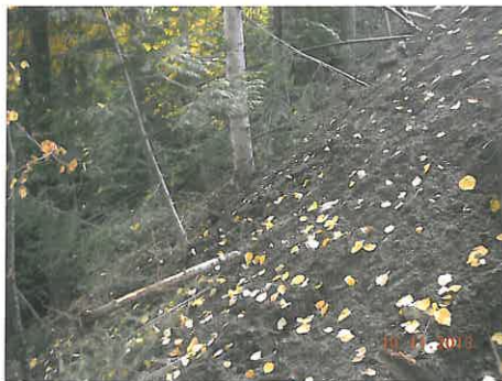
Photo 6 above: View of the temporary access trail under construction, during initial preparation for slide repair. As the temporary slope height exceeded 6 m, a written "safe entry" protocol was developed by AMEC under which Gibraltar's staff was conditionally granted access to work in the excavation. The large boulders in the photo were scavenged from the existing embankment fill and were incorporated into the lower "stack wall" part of the embankment repair. The inset view shows the temporary stockpile of rip rap armour which was obtained from Mt. Polley. Photo 7 upper middle: View looking upslope in the scour channel developed below the slide, at the toe of the new embankment. The boulders were placed individually on a prepared base and interlocked at a nominal 40-45° slope. The inset view shows the scale of some of the larger rip rap blocks placed at the slide toe. Photo 8 upper right: Panoramic view looking downslope at the former slide area, from the restored road shoulder. The dashed line marks the approximate transition from larger placed rip rap, and more variably sized angular rock (both from Mt. Polley and from the rock slope area at the site). The inset is a closeup view of the flow channel below the slide. Some rock chunks came loose during placement, and came to rest a short distance downslope in an area of irregular bedrock exposed in the debris channel created below the slide zone. The rocks are interlocked and are considered to be stable. Photo 9 lower left: View looking downslope across the restored road fill embankment. The dashed lines mark the approximate location of the temporary access trail. The red arrow points to the approximate location of loose fills dispersed downslope into the forest during trail construction (see Photo 10). Photo 10 lower middle: View looking easterly across the fill materials on the ground surface downslope from the temporary access trail. The slope of the fill is approximately 38°. Photo 11 lower right: Panoramic view looking up/westerly along the restored roadway and fill embankment area at the slide repair site.
