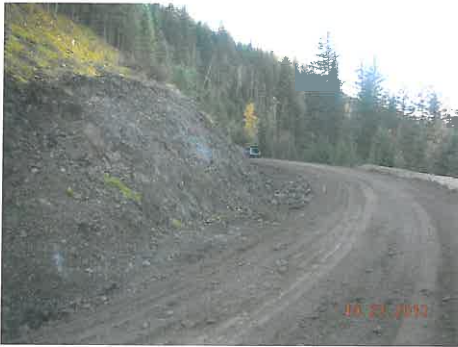
Photo 1 above: Preconstruction view looking west/upslope along the roadway segment adjoining the rock bluff. Note the obstructed sight lines at the road corner, lack of a ditch line/debris catchment area along the slope toe, and infilled/outwards leaning barrier elements. Photo 2 upper middle: view from a similar location after construction. The rock slope toe area was trimmed to establish a ditch/debris catchment area along the slope toe, and vegetation was removed from the lower part of the slope. Note the concrete guardrail blocks (photo centre) were lifted and re-seated on a low fill embankment. The window of gravel along the guardrail created during grading was removed after the photo was taken. Photo 3 upper right: closeup view of the east/downslope end of the rock slope toe area which was reconfigured by Gibraltar. Photo 4 lower left: View looking westerly "around the corner" at the west end of the rock outcrop area. Note the improved sight lines along the corner, and ditchline established at the slope toe. Photo 5 lower middle: View looking easterly/down the road, at the central part of the rock slope which was trimmed. Note the clearing/removal of vegetation above the crest of the cut slope. Ideally, small trees which become established in this area should be removed from time to time, to prevent them from growing to mature size to the stage they may become a hazard to road users.
