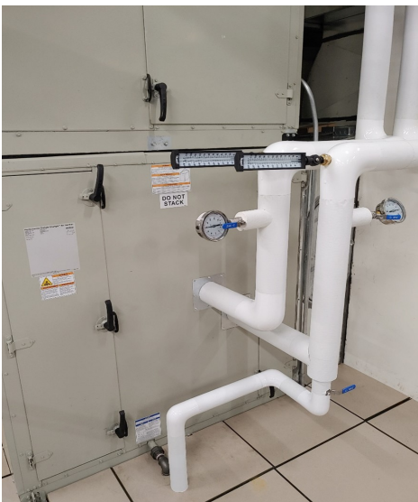
Figure 2: Server Room Cooling Coil
