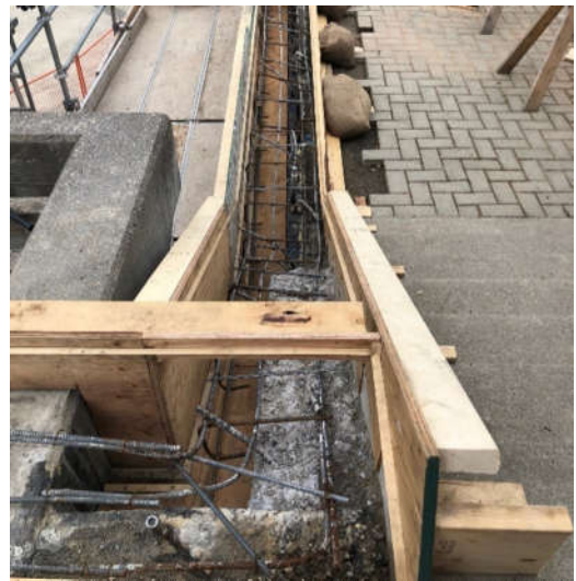
Doug Little Lounge – Concrete Restoration: Formwork and rebar ready for pour of new concrete
