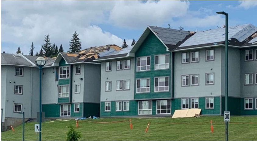
Residence 1 Roof Replacement: Original shingled roof was installed in 1995, replaced with new shingles in 2022.
