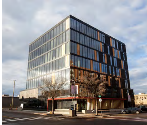
Figure 2.18 Wood Innovation and Design Centre
