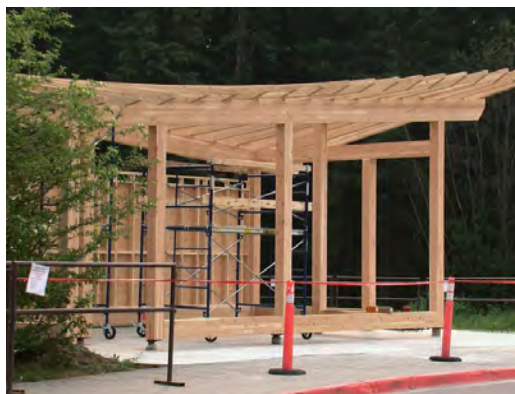
Figure 2.9 UNBC Bus Shelter Under Construction
