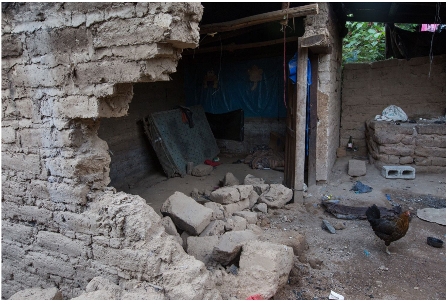
An abandoned home in La Cuchilla, that crumbled and partially caved in due to tremors caused by the use of explosives in Tahoe's tunnels. San Rafael Las Flores municipality, Guatemala.
