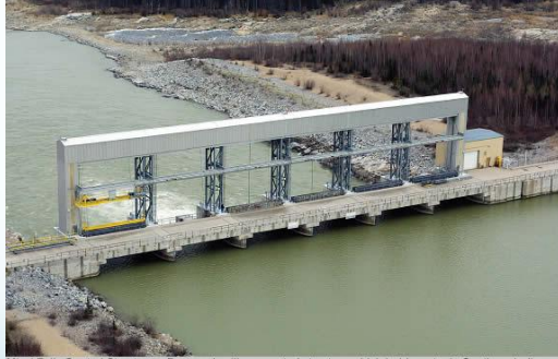
Missi Falls Control Structure – Dam and spillway control structure which holds water in Southern Indian Lake and regulates the volume of water passing down the lower Churchill River.
