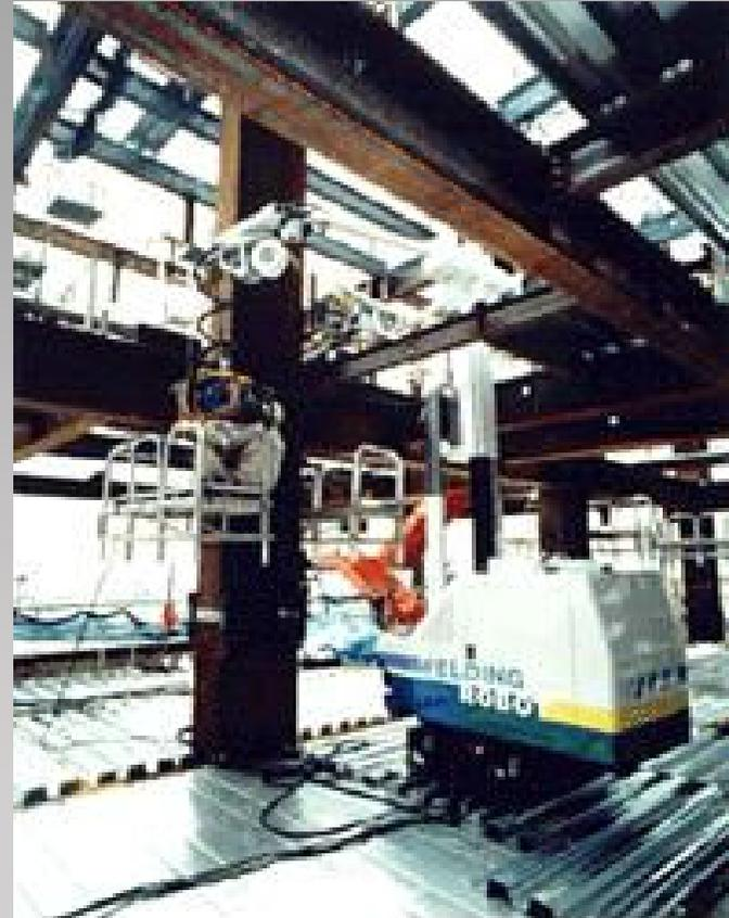
Welding robot installed
