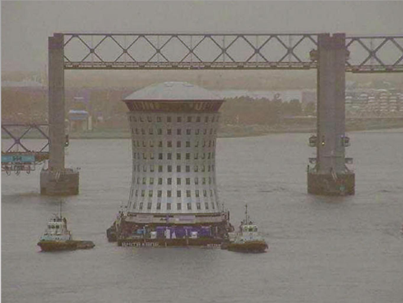
10 story Steel and glass office tower manufactured in a ship building yard in the Netherlands
