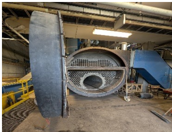
Down for annual maintenance. The "Fire Tube Boiler" heats up our Campus water. It's open so the tubes can be cleaned & punched. Once the ash is cleaned out, the "Fire Tube Boiler" is ready for inspection.
