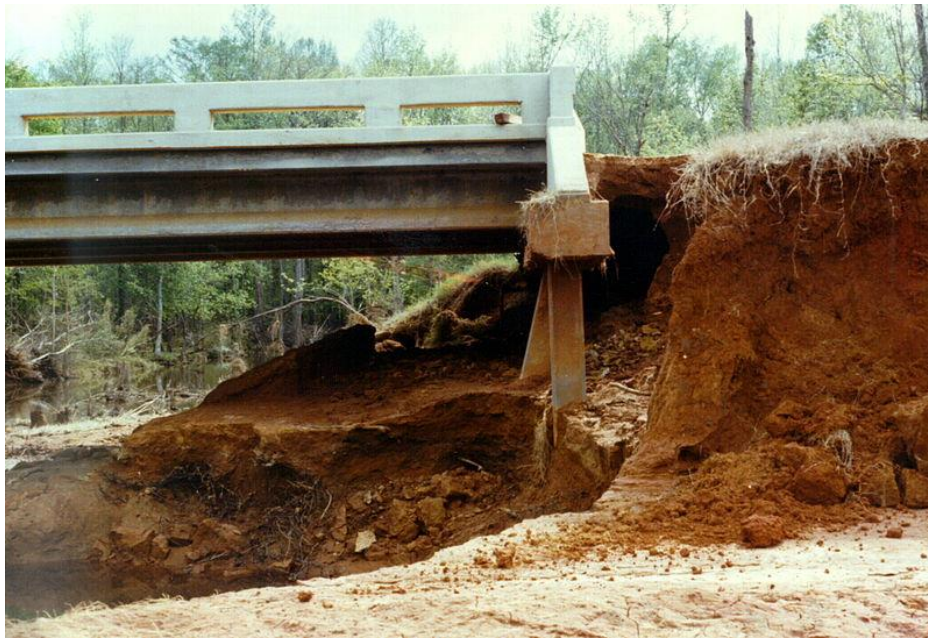
Figure 1- 1 A typical local scour around a bridge abutment
