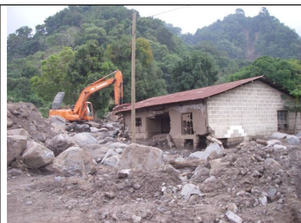
Figure 7. Digging out in a rural community south of San Lucas Toliman
